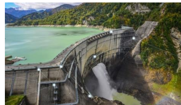
Structural Health Monitoring
